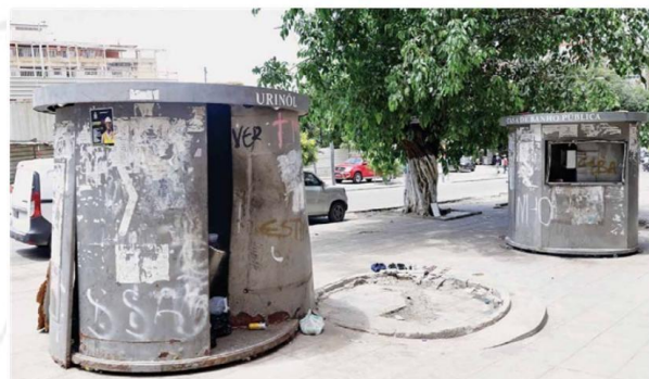
FIG 136: DUE TO LACK OF MAINTENANCE, PUBLIC TOILETS IN WORTH SEVEN MILLION USD OF INVESTMENTS FROM LUANDA'S PROVINCIAL GOVERNMENT WERE REMOVED FROM THE STREETS OF DOWNTOWN LUANDA IN JANUARY OF 2024. PUBLICATION IN A LOCAL NEWSPAPER, NOVO JORNAL, OF JANUARY 20TH, 2024.
