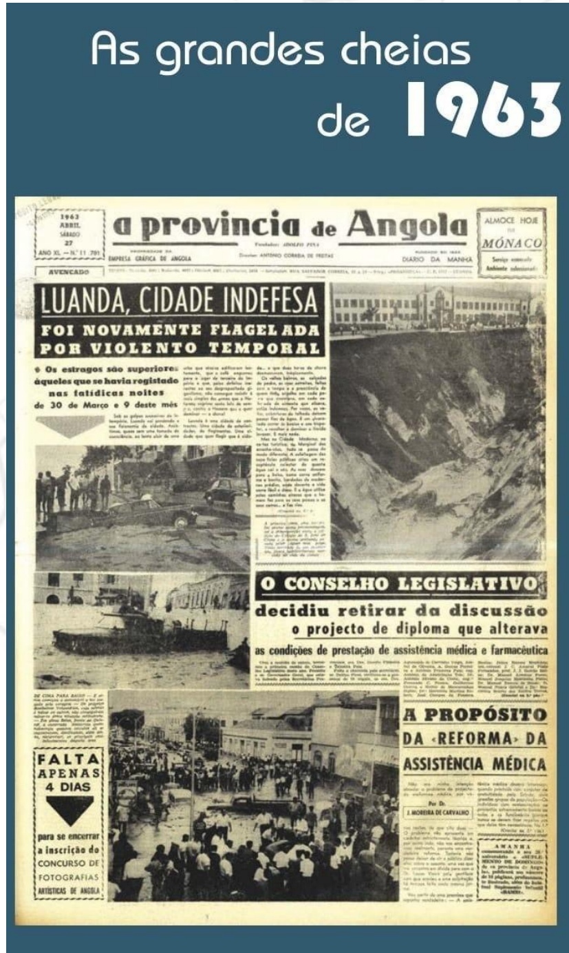
FIG 1: A JOURNAL PAGE SHOWING THE DAMAGE CAUSED BY OF HEAVY RAINS IN LUANDA IN 1963 SOURCE: GARCIA, 2016, P. 132
