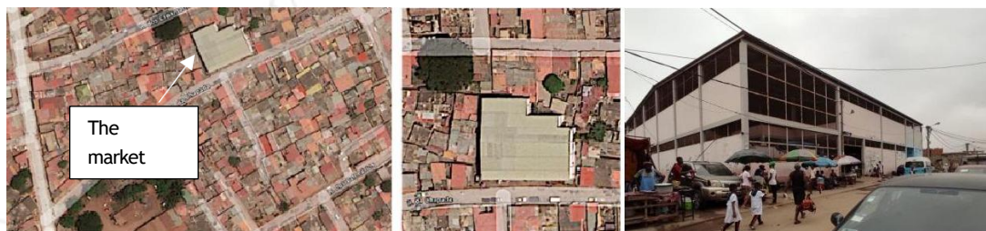
FIG 25: PHOTOS ILLUSTRATING THE DENSE CONTEXT WHERE MERCADO DA CHAPADA IN LOCATED IN MARÇAL AND A PHOTO OF THE EXTERIOR OF THE BUILDING FROM THE ONLY ACCESS IT HAS NOW. PHOTOS TAKEN IN JUNE 2021. SOURCE: LURA ARCHIVES, 2021
