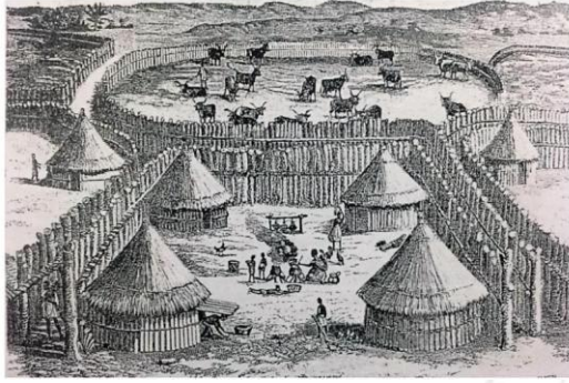
FIG. 16: DRAWING FROM 1888, REPRESENTING A FAMILY DWELLING IN A VILLAGE IN HUNDE, NAMIBE PROVINCE IN THE NORTH OF ANGOLA.
