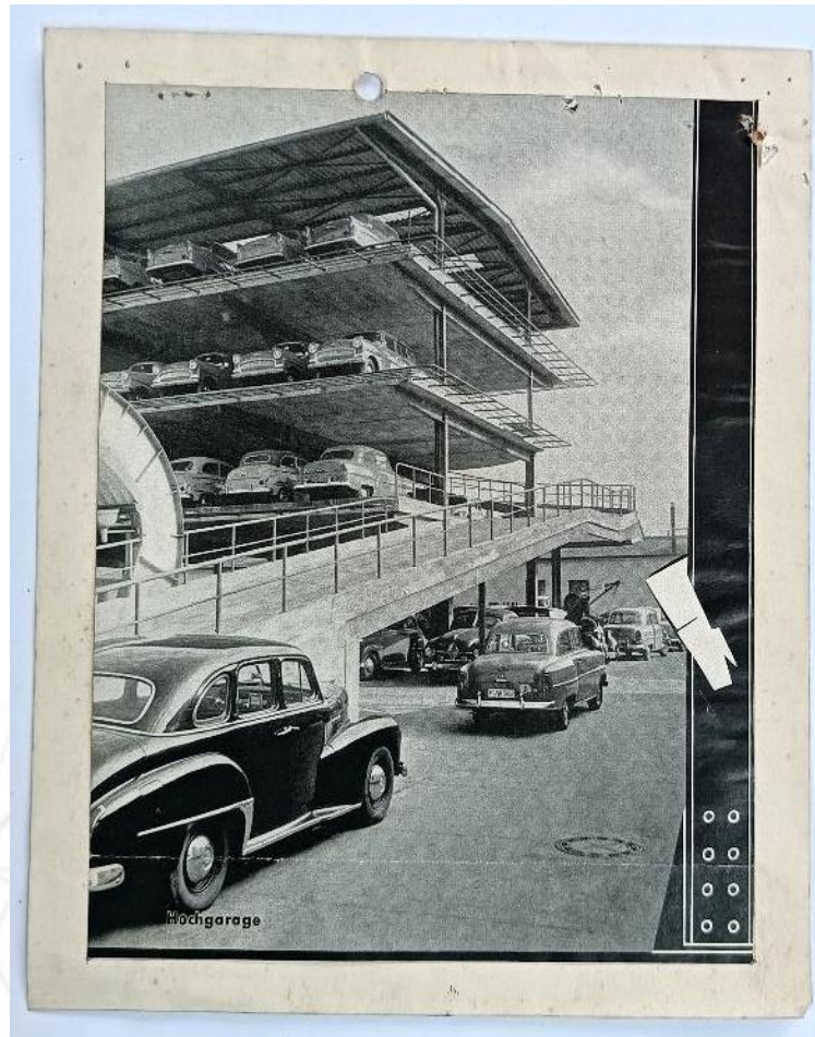
FIG 3: A PHOTOGRAPH OF THE VERTICAL PARKING FACILITY, PROPOSED FOR CONSTRUCTION IN MUTAMBA, NEAR DO CARMO'S PARK, WHERE A MULTIMODAL JUNCTION CONNECTING THE CITY CENTRE TO THE BAY WAS ALSO PROPOSED.
