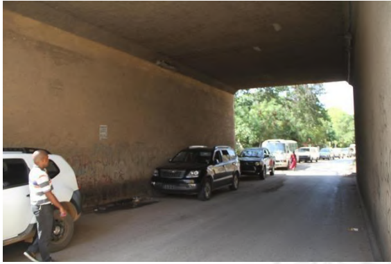
FIG 39: NAXIXI STREET BEFORE INTERVENTIONS IN 2020
