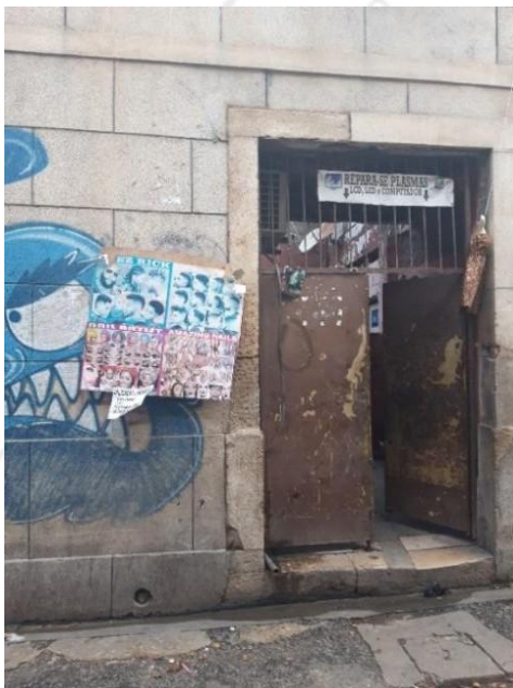
FIG 35: PICTURE OF A PORTION OF RUA DOS MERCADORES WITHOUT INTERVENTION.
